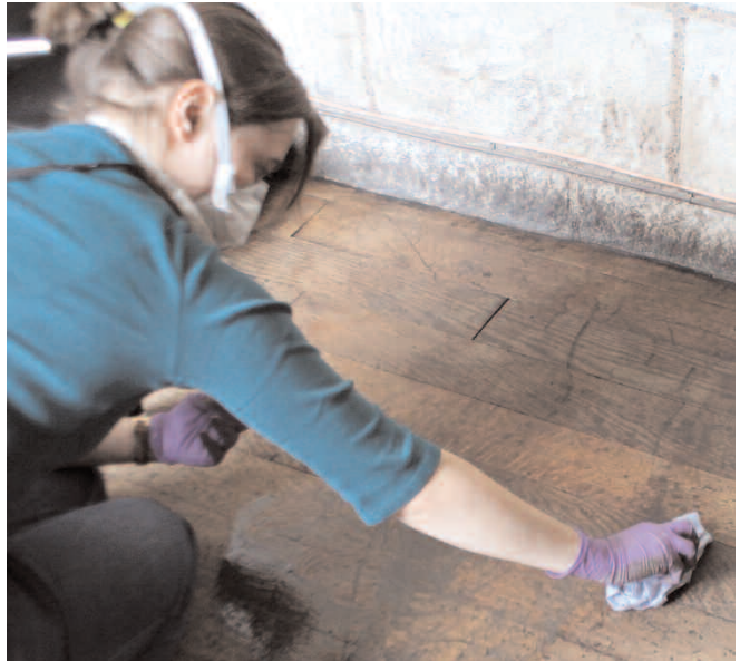
Rhian, the conservator removing the shellac varnish from the Tunstall Gallery floor.
